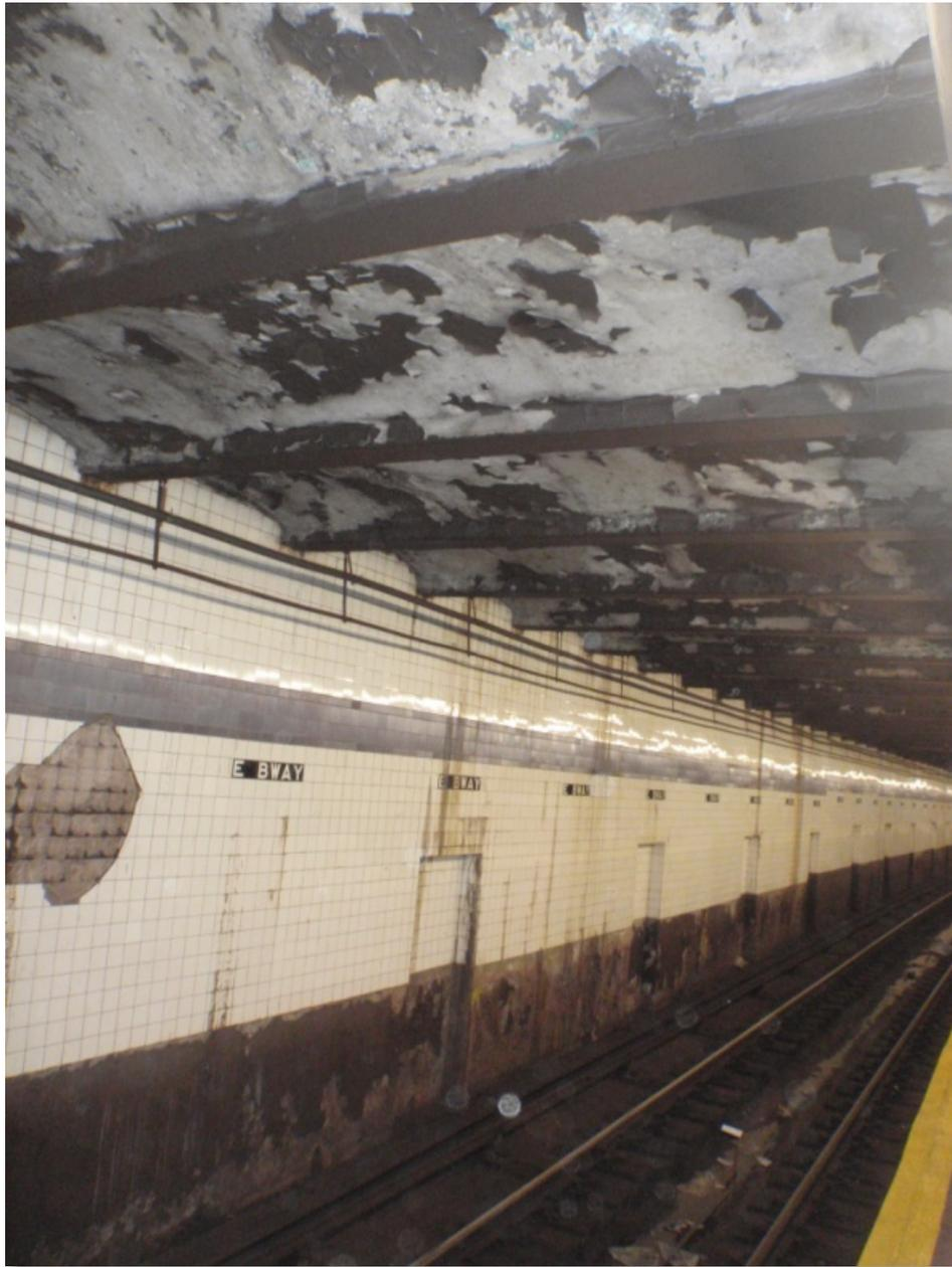
A) Excessive peeling paint on ceiling over track. (Photo taken on 3/14/14)
